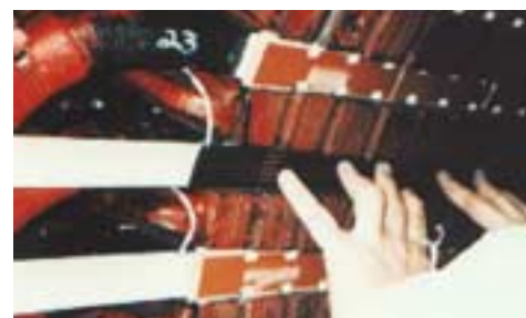
Stator Slot Coupler Installation
